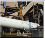
TAI provided services for the installation of outdoor Urea Storage Tank foundations, chemical containment, and integration of the Advanced Combustion Technology (ACT) skid units into the plant mechanical, electrical and control systems. Additionally, TAI provided design engineering to route piping and cabling between skids and from the Urea storage tanks to the distribution headers and injectors.
