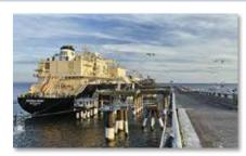
The Client aimed to further develop the infrastructure to increase the ship unloading capacity from 155,000 cubic meters of LNG to 267,000 cubic meters of LNG. TAI was brought on to reinforce the offshore platform to
