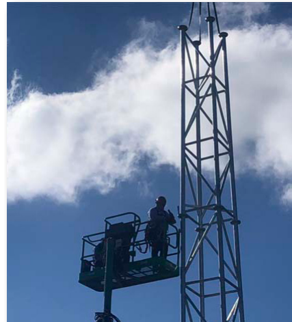
Operator bolts assemblies into place.
