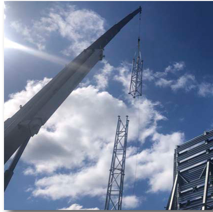
Cranes lift piece number 4 of 5 in place.
