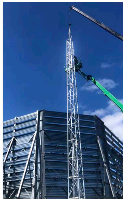
Final piece of tower secured in place.
